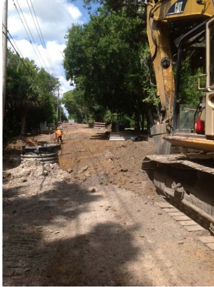
Photo No. 1 – Road excavation in the 500 Block of Hand Avenue.
