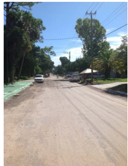
Photo No. 2 – Preparation to pave east of Center Street.
