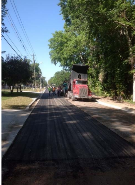
Photo No. 1 – Paving of the 600 block
